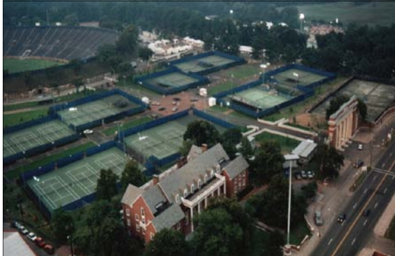
Connecticut Tennis Center at Yale University New Haven, Connecticut
