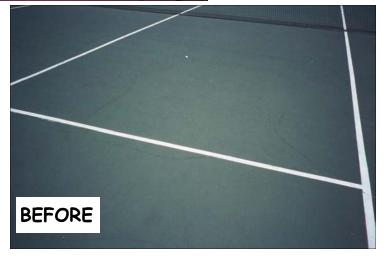
These twelve tennis courts were constructed in 1976 with the WESCO emulsified asphalt leveling course system of construction. The courts endured well until 1997 when the University decided to rehabilitate the courts and redesign the lighting system to improve the safety for the players. Drainage was added and the slope of the courts increased to improve the drainage. Global was engaged to provide the rehabilitation expertise.
