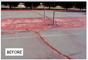
These tennis courts at Sandy Brook Park were unusable and unsafe due to the aging and cracking of the asphalt leveling course. It was determined that pulverization of the existing pavement and its reuse as an aggregate base course would be the most economical approach to the court rehabilitation.
